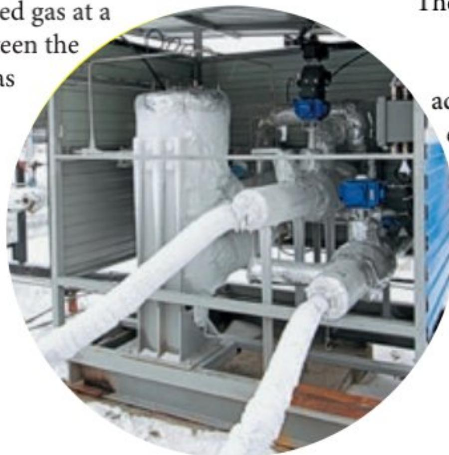
The concept was based on the principles of the maximum possible use of secondary energy sources, which are, in fact, energy losses during the main gas transportation. Russian engineers managed to find a way to use them effectively by using a turbo expander.
